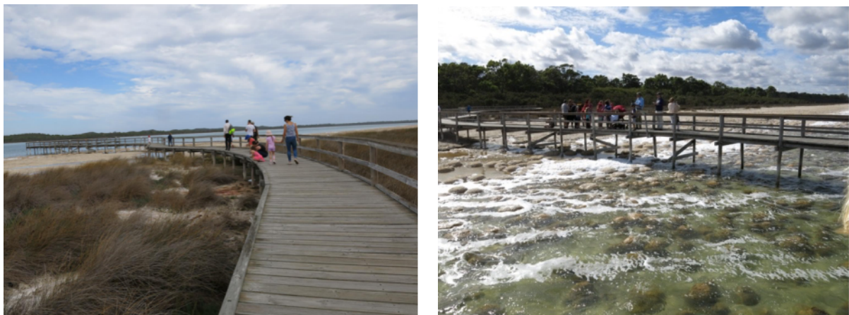
Figure 6a & b. Boardwalk
